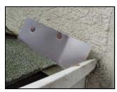
A functional kickout flashing can NOT be mounted on top of the cladding.
