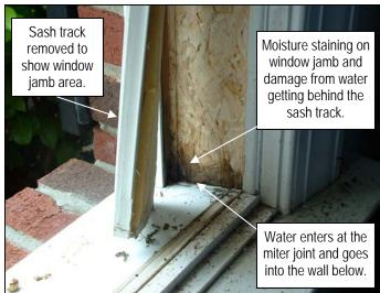
This is a photo of the miter joint behind the plastic sash track on a double hung window. Moisture that gets behind the sash track can drain directly into the wall cavity.
