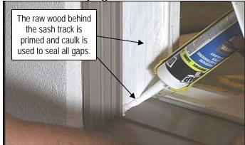
This is a photo of a double hung window with the sash track removed. When properly primed and sealed, the miter joints of windows can be successfully repaired and will stop most leaks.
