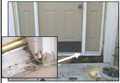
Door leaks are similar to leaks at windows. The corners (miter joints) commonly have openings that leak. The threshold of the door may also be leaking. Modifications to the door must be made to stop these leaks. Framing below the door may require repair.
