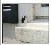
Wood Rot: Rotted areas must be repaired or replaced.
