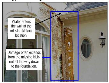
Because significant amounts of water can enter the wall at a missing or improper kickout location, severe damage is possible. Most homes have an average of 4 kickout locations, at least one of which is usually leaking.
