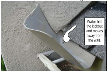
A MoistureFree approved kickout flashing is a pre-engineered, weather tolerant plastic flashing that fits behind the last piece of step flashing. The brand name is Raintec® and is easily available to all repair contractors. Make sure that your contractor uses only a MoistureFree approved kickout flashing on your home as others are oftentimes unreliable.
