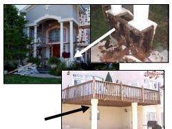
Support columns on decks and entry ways are often missing flashing and sealants.
