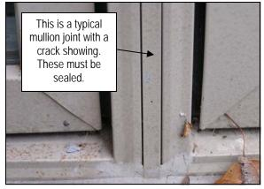
The mullion is the joint between sets of window units. Openings in the mullion joint can allow moisture to enter
