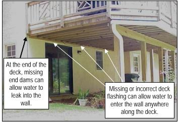
Most decks are attached directly to the framing of the home. The joint where the deck is attached must be flashed to protect the wall below. End dams are required to stop water at the edge of the flashing from flowing into the wall.
