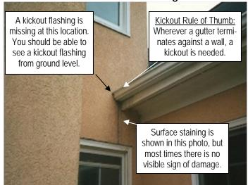
A kickout flashing is a flashing that directs water away from the home and is located where the roof edge terminates against a vertical wall. If the kickout flashing is missing or installed incorrectly, water from the roof can run directly into the wall cavity.
