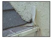
Hand or field made kickouts fail at a very high rate.
