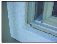
Failing Caulk: The correct type of caulk and proper installation of the caulk is required.
